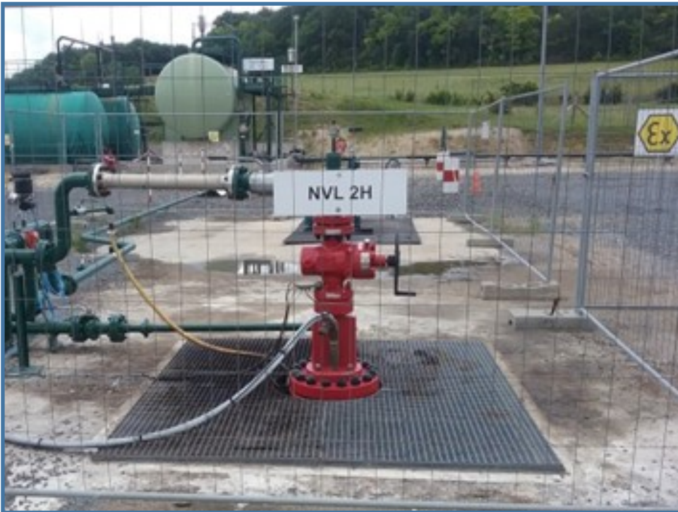
Photograph of the wellhead for well NVL2H, equipped with an ESP (Nonville site).
